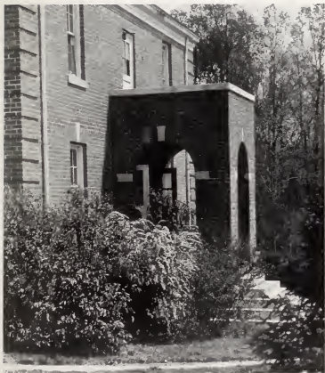
WEST ENTRANCE, WHITAKER HALL
