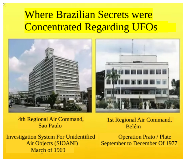
Fig 2.6 – 4 th Regional Air Command Building & Operation Prato In The 1 st Regional Air Command Building
