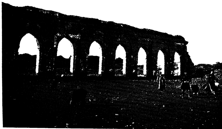
FIG. 38.—RAQQAH, ARCADE OF MOSQUE, FROM NORTH.
