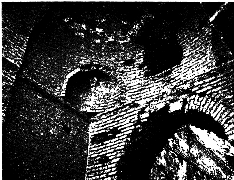
FIG. 154.—SÂMARRÂ, BEIT EL KHALÎFAH, DETAIL OF VAULT OF SIDE CHAMBER
